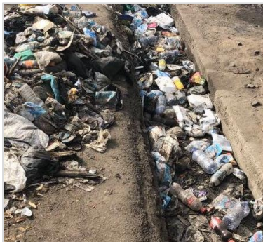
Drainage system in Agbogbloshie, Accra
