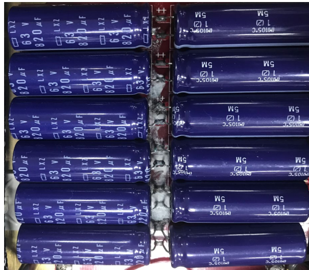
Figure 15.3. Capacitor damage within the side-scan sonar unit prior to repair.
